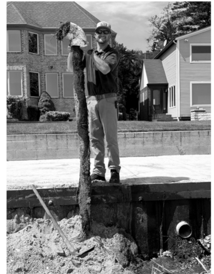
Marvin had to dig up and replace the line to get rid of this root mass.
