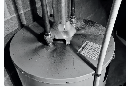
Rust stains and melted plastic grommets on the top of a water heater are tell-tale signs of a back drafting water heater.
