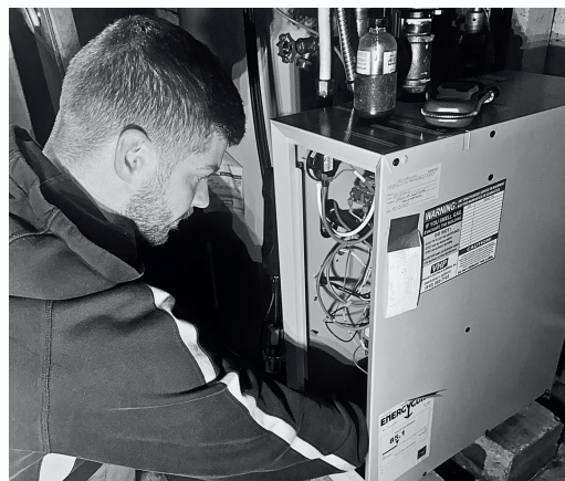
VHP tech Nathan performing annual service on a hot water boiler. This provides peace of mind and savings for our Enhanced Service Plan clients.
